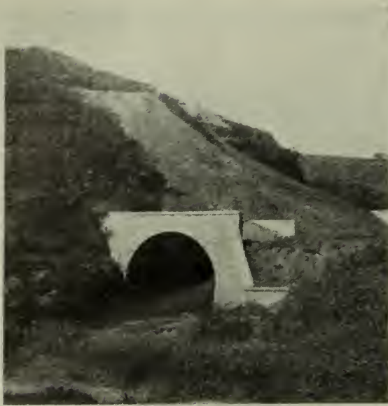
FIG 3.—UPSTREAM ENTRANCE TO STERKSPRUIT CULVERT.
